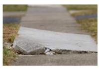
change in walking surface of Month 1/4" or greater is sufficient to cause a trip. Curbs, sidewalk cracks, bumps, potholes,
